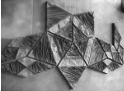
(a) Exterior wall
